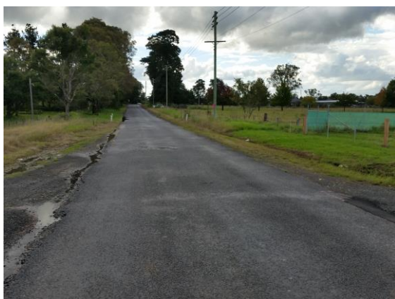
Great Southern Road, looking N
